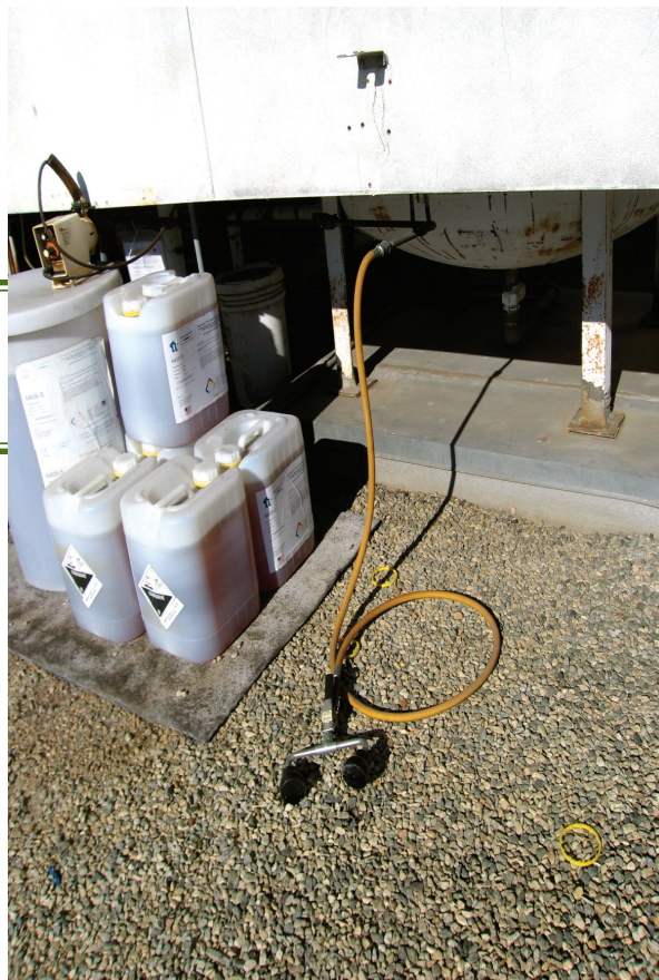
Eyewash station with potential hazardous material
