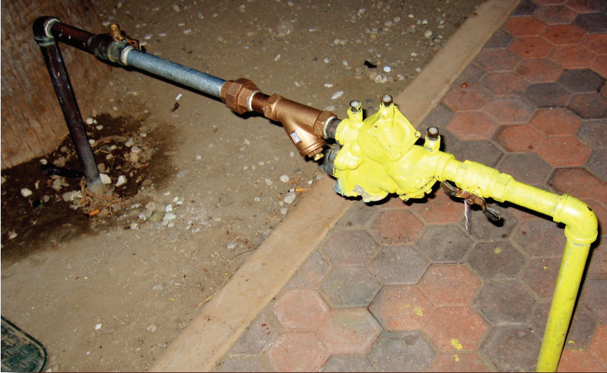
Strainer incorrectly installed downstream of the No. 1 shutoff valve, but upstream of the body of the backflow preventer
