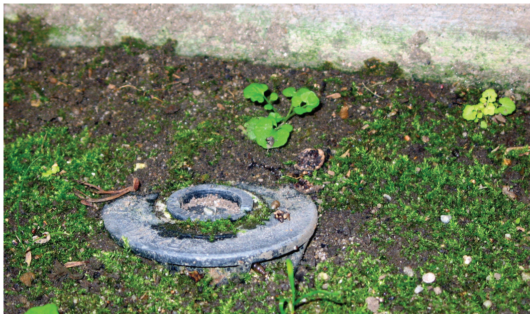
Pooling around sprinkler head that may contain hazardous material
