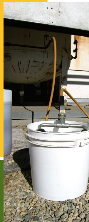
Eyewash submerged may contain hazard
